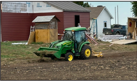
Extensive grading was done on the Wheels grounds this past year.
